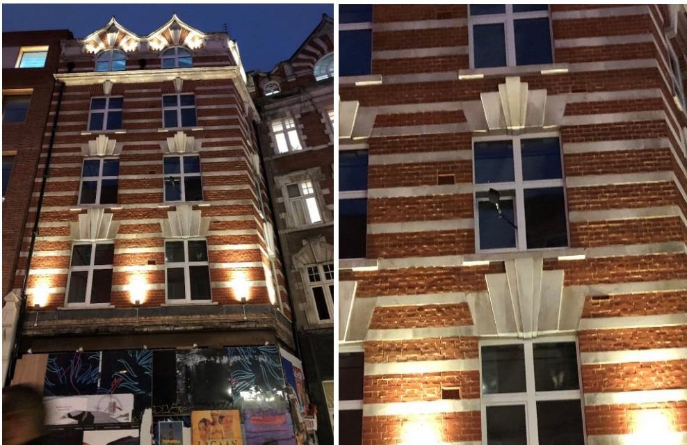
Figure 2 Unattended logger position
